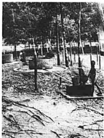
Plate 50. Estate sanitation. Water supply was drawn from brick wells. Contamination was prevented by enclosing the wells within a barbed-wire fence. The water was drawn by a pump on Tremelbye Estate, Federated Malay States ( Source : Arkib Negara Malaysia).
