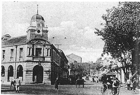
Plate 35. The Kreta Ayer Jinrikisha Branch Office c. 1906. This establishment was opened in 1904; it replaced an earlier building. It was used for licensing jinrikisha vehicles. It is situated at the junction of Tanjong Pagar, Neil and South Bridge Roads (Source: National Archives, Singapore).
